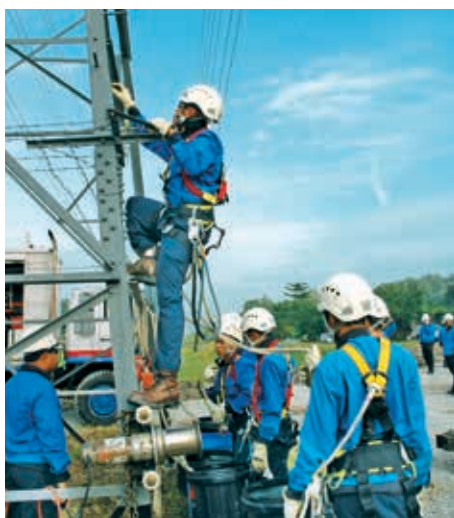
Tenaga Nasional technicians conduct maintenance work at a power transmission tower
